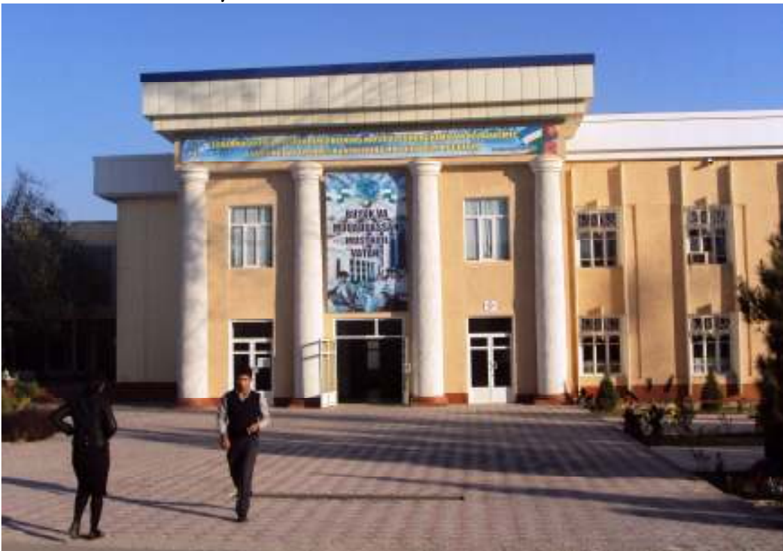
Main entrance inside the yard
